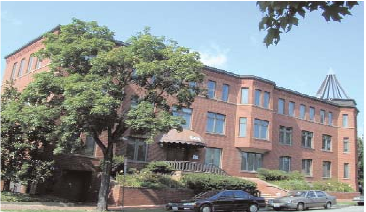
CAIR acquired this building two blocks south of the Capitol to serve as its main headquarters.
